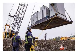
When sites are not accessible with a trailered unit, IMG substations are assembled on a rigid, steel skid typically consisting of 8x6" tubing skid, point-of-connection for tow/lift hooks, grated floor for non-skid, and oil-containment where required. Outdoor-type enclosures are used for Incoming & Outgoing sections to protect equipment from environmental elements.
