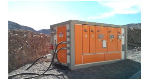
Features include Arc Flash metering & protection, visual indicators, and physical barriers that protect against damage to equipment and personnel.
